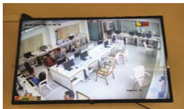
LED Screen for CCTV Display
