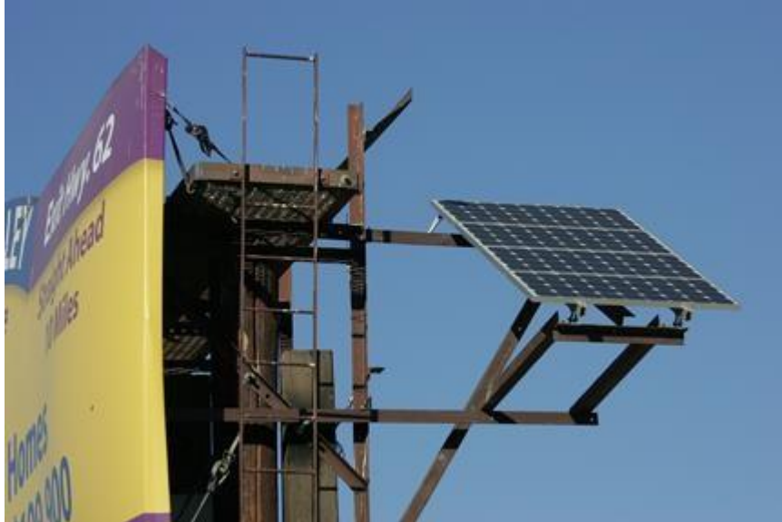
Figure-1: Solar powered light for Hoarding
